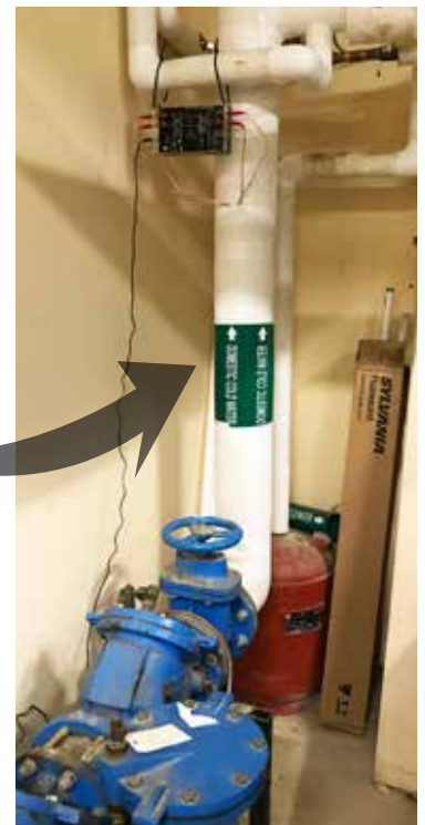
Step 2: Install the S25 unit on the water main and wrap the protection layer
