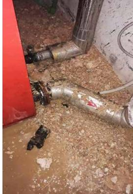
The scale deposits were easily removed The scale deposits were drained out of the boiler with ZERO chemical.
